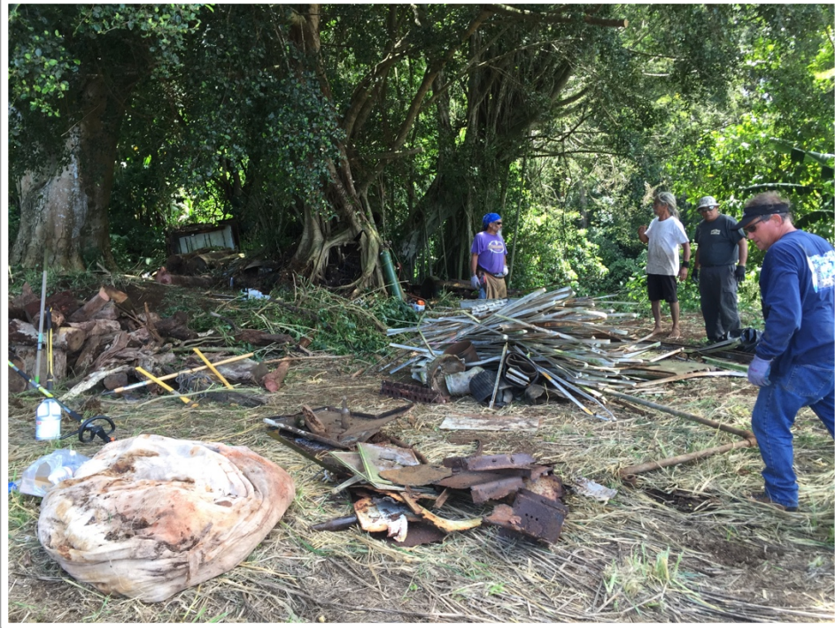
Metals that were pulled out, loaded and hauled away.
