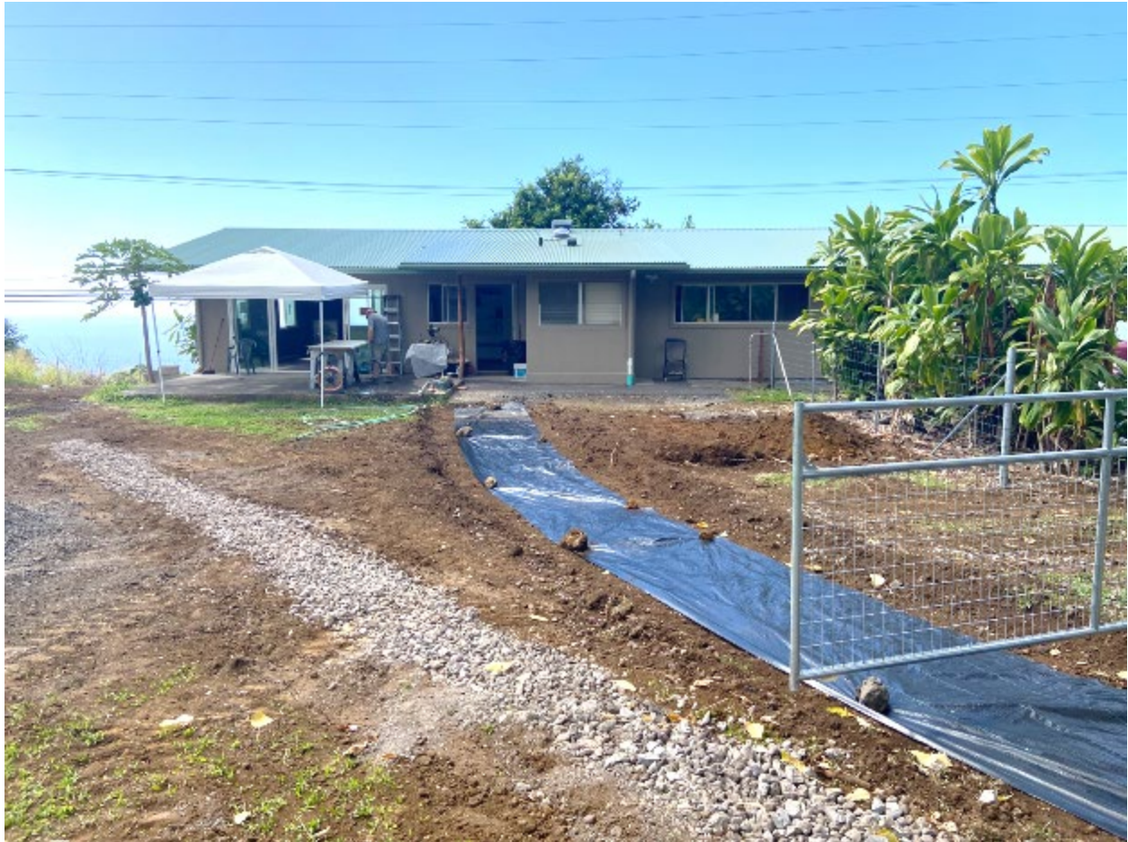
Figure 2. The newly renovated exterior of the former Amy Greenwell residence. Trees and brush have been removed, the new pathway has been designed, and the exterior walls have been painted.
