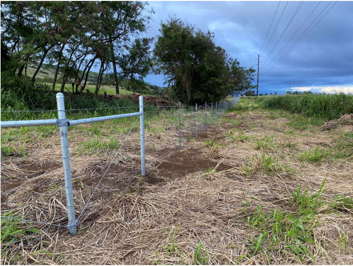
New Fence Along Highway, View to East – April 01, 2020
