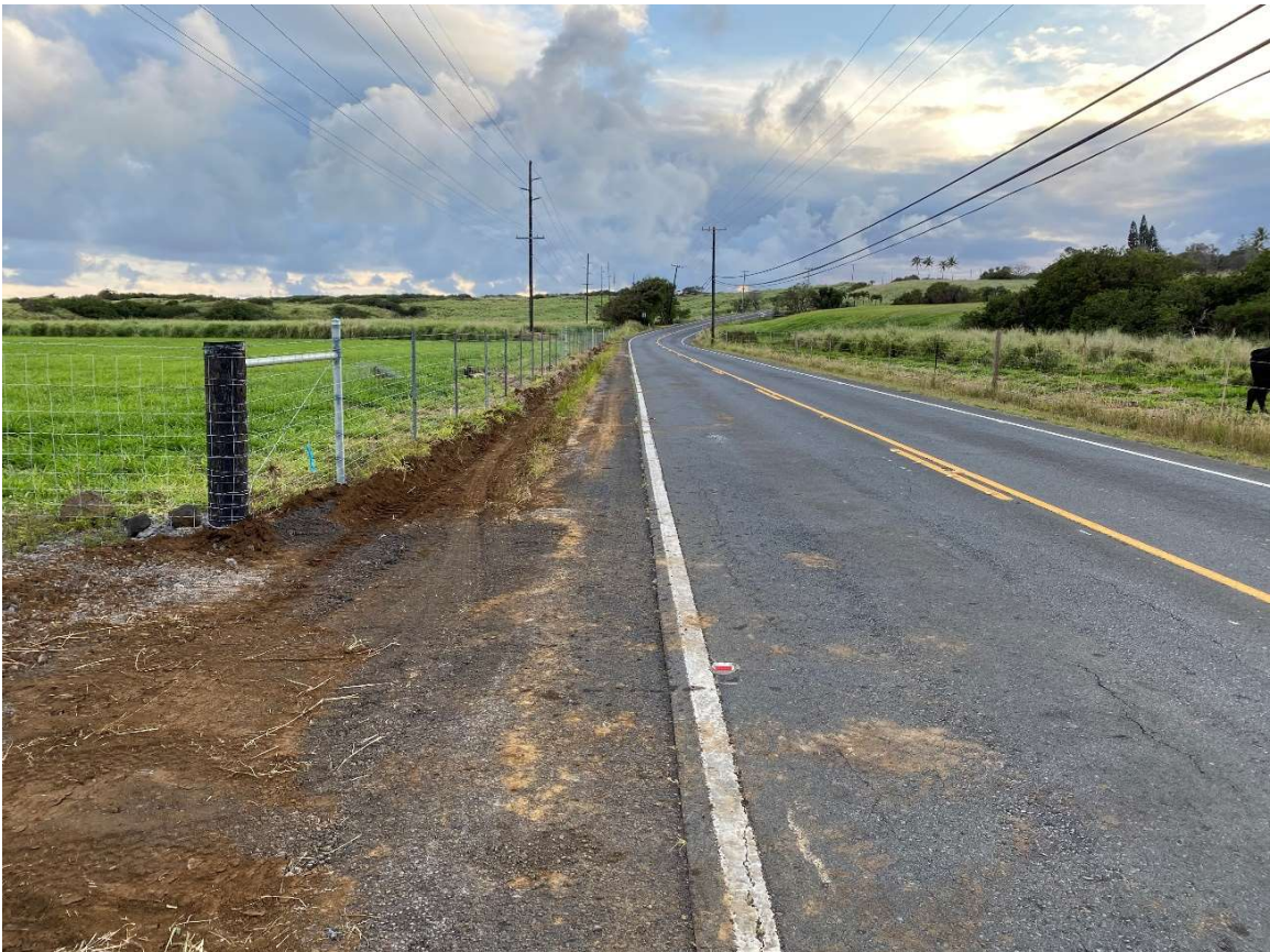
New Fence Along Highway, View to West – April 01, 2020
