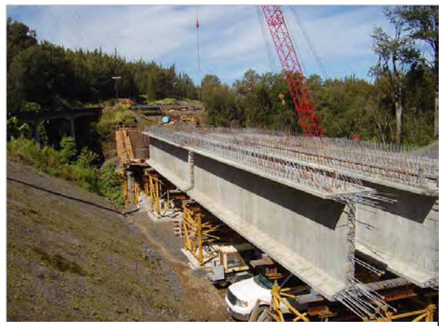
Kealakaha Stream Bridge Replacement, Hawaii (2010) Construction Cost: $36M
