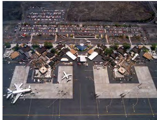
Various Construction Projects, Kona International Airport (1998-2009)
