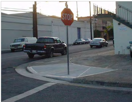
RMTC assisted the State Department of Transportation, Highways Division, with management of the highly-expedited design and construction of over 1,600 curb ramps statewide. Total cost of the project exceeded $22.1 million.
