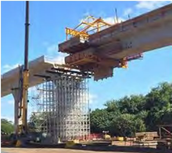
Typical rail guideway section under construction from East Kapolei. Jacobs managing the environmental compliance and coordinating activities under the historic preservation program.
