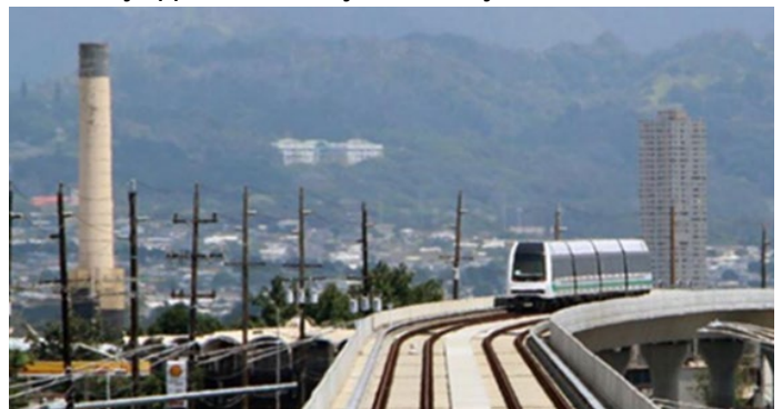
Typical elevated rail guideway section in Waipahu
