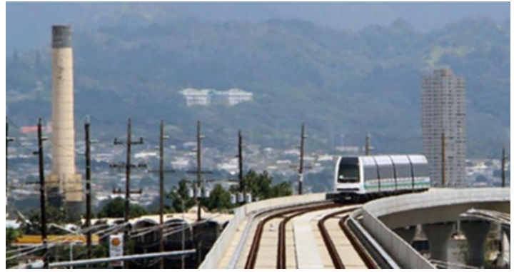
Typical elevated rail guideway section in Waipahu
