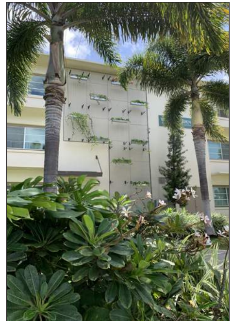
Planter Box Wall Installation
