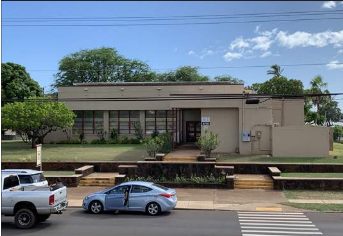
View of Solar Panels Atop Building
