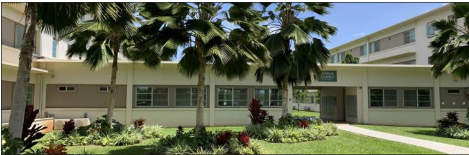
Entry to Front Office
