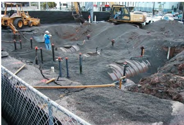
UST closure excavation at Kaneohe Chevron Service Station
