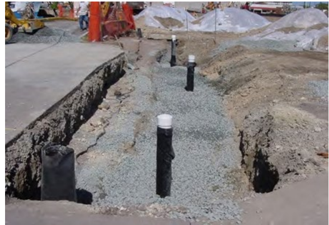
Installation of subsurface barrier and intercept trench at Pier 35
