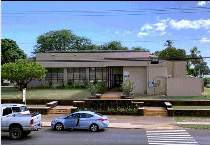
View of Solar Panels Atop Building
