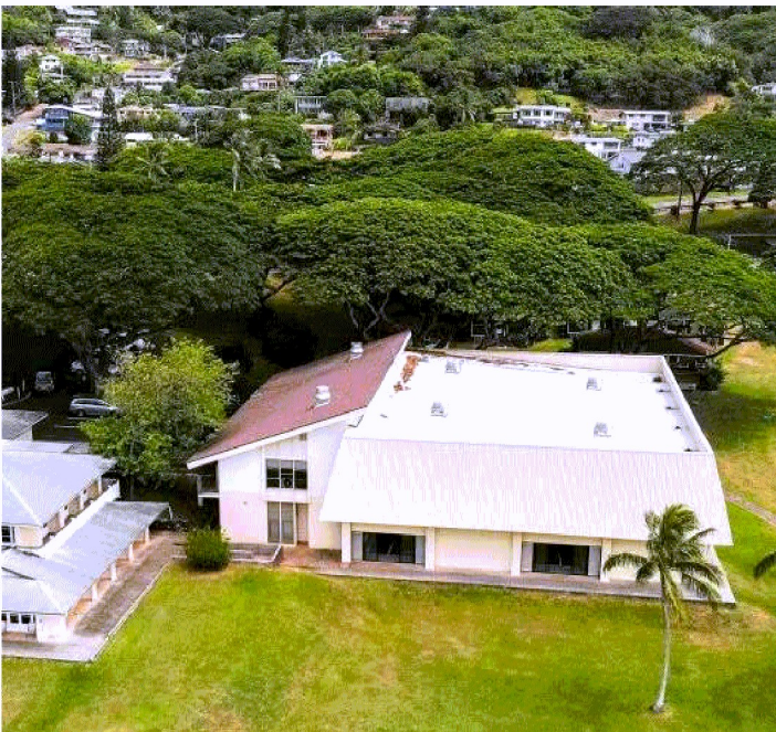
AERIAL IMAGE (Gym at Right)
