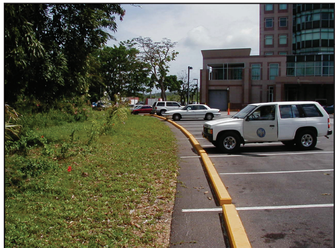
Figure 1.6 Use of a Grassed Filter Strip.
