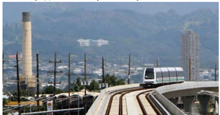
Typical elevated rail guideway section in Waipahu
