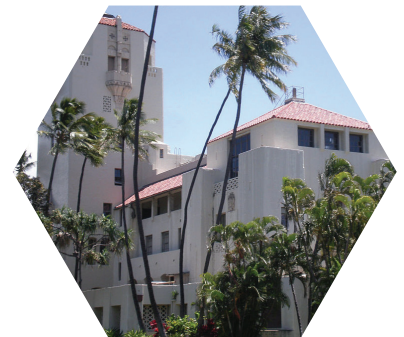
Construction Management Services for City Hall Fire Alarm System Improvements
