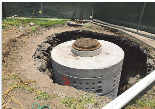
Seepage pit installation at Nani Olu
