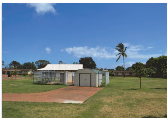
Completed treatment system site
