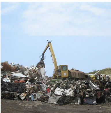
We provided our client with a cost-effective way to test for lead in approximately 44,100 cubic yards of soil and debris.
