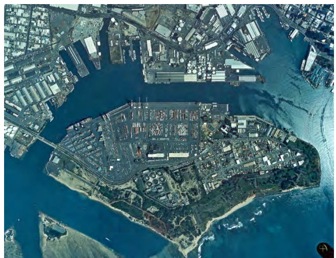
RMTC has designed over $500 million in harbor infrastructure throughout the State of Hawaii.
