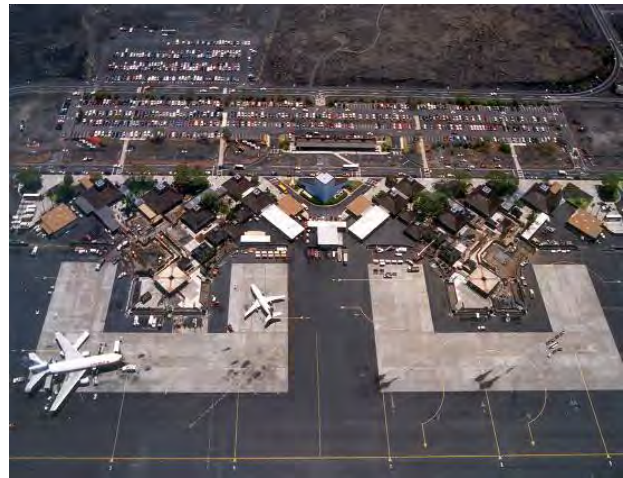
Various Construction Projects, Kona International Airport (1998-2009)
