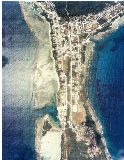
RMTC prepared an engineering planning study for flooding and drainage problems within Sinapalu Village on the Island of Rota. The hydrologic and hydraulic analyses were performed to identify flood hazards within the village.
