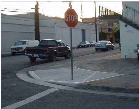
RMTC assisted the State Department of Transportation, Highways Division, with management of the highly-expedited design and construction of over 1,600 curb ramps statewide. Total cost of the project exceeded $22.1 million.
