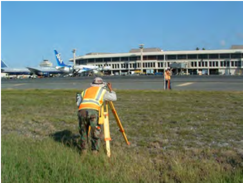
RMTC surveyors perform a topographic survey at the Daniel K. Inouye International Airport, Oahu.
