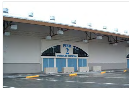
Pier 2 Cruise Terminal, Honolulu Harbor, Oahu (2006)
