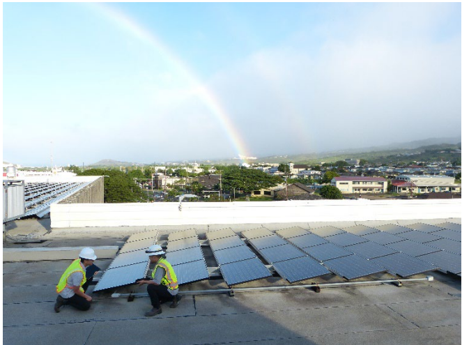
Inspectors check layout of PV modules
