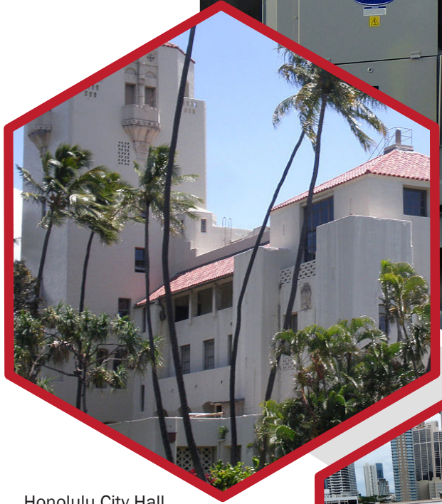
Honolulu City Hall Fire Alarm System Improvements
