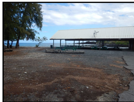
Miloli‘i Beach Park – Existing Conditions of Parking Lot and Pavilion
