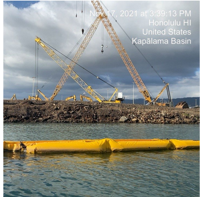
Demolition work within Snug Harbor
