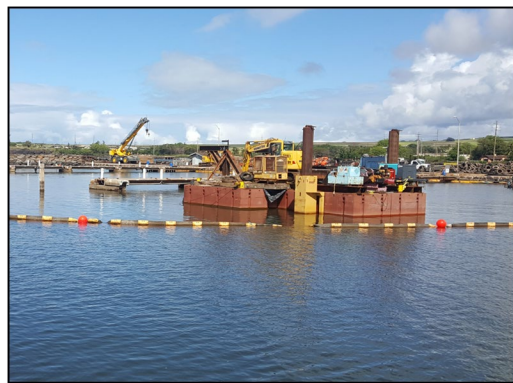
Turbidity curtains are shown around the in-water work area
