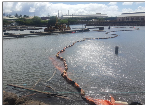
Turbidity curtains installed around the harbor
