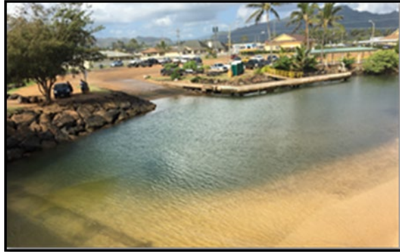
Sand accumulation visible near the boat launching area
