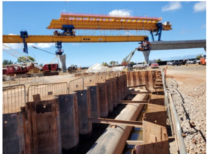
Jacobs maintained operation of the WWPS while constructing a major pipeline through reclaimed land and coordinated with ongoing construction along the alignment.
