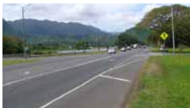
Kahekili Northbound Approach at Ahaolelo
