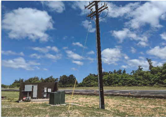
Electrical service upgrades
