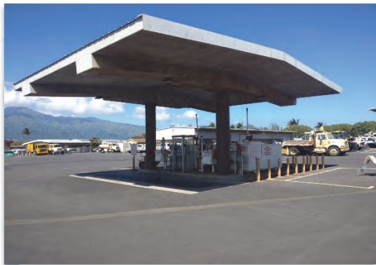
Existing fueling station
