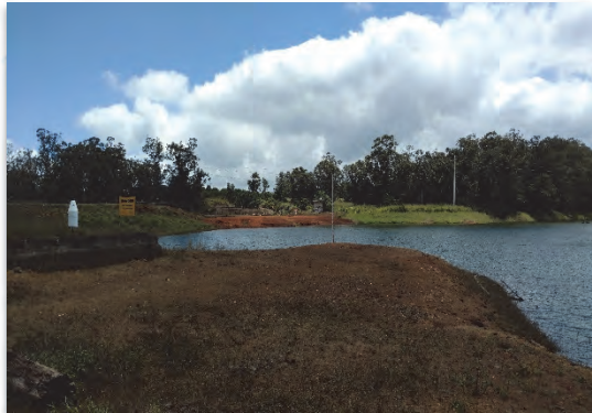
Dam Spillway at the Wahiawa Reservoir
