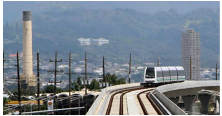
Typical elevated rail guideway section in Waipahu
