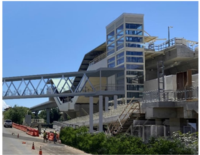
Pearl Highlands Station with pedestrian bridge over Kamehameha Highway
