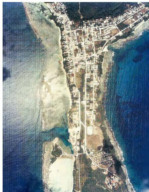
RMTC prepared an engineering planning study for flooding and drainage problems within Sinapalu Village on the Island of Rota. The hydrologic and hydraulic analyses were performed to identify flood hazards within the village.
