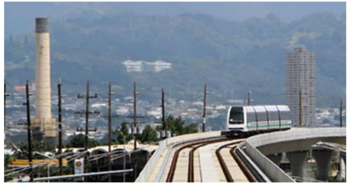
Typical elevated rail guideway section in Waipahu
