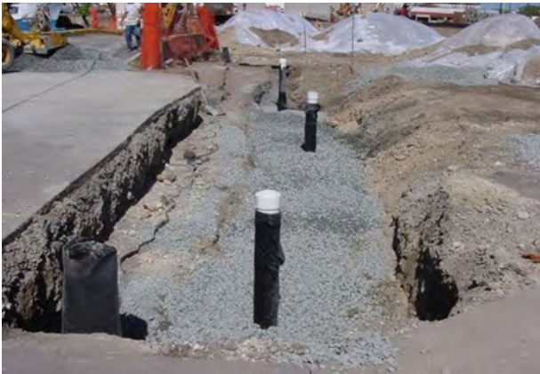
Installation of subsurface barrier and intercept trench at Pier 35
