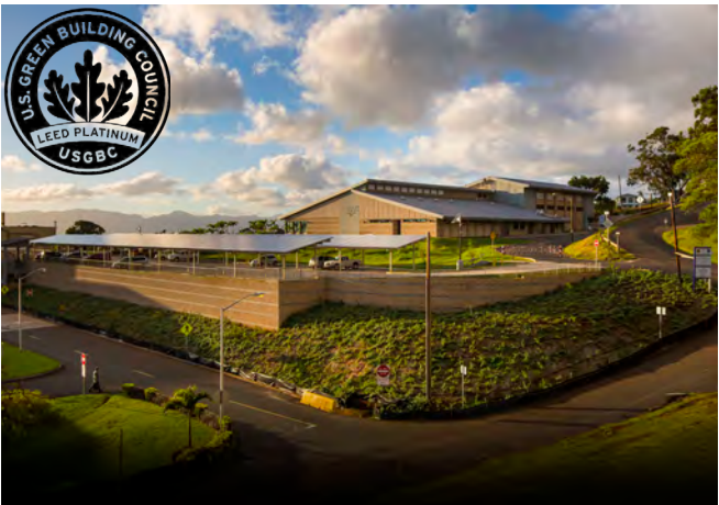
Camp Smith Physical Fitness Center (LEED Platinum)
