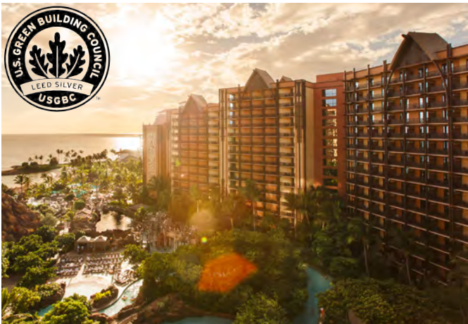
Aulani, A Disney Resort & Spa (LEED Silver)
