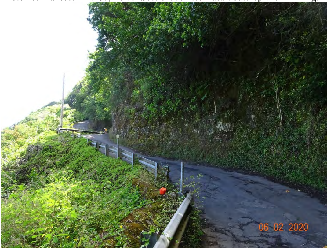
Photo 18. Transect F-W-07, Lower Section. Note small deformed retaining wall makai side of road.
