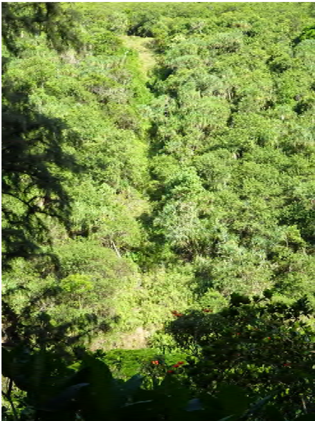
Photo 30. Waipi‘o Valley Road slide area from beach road.
