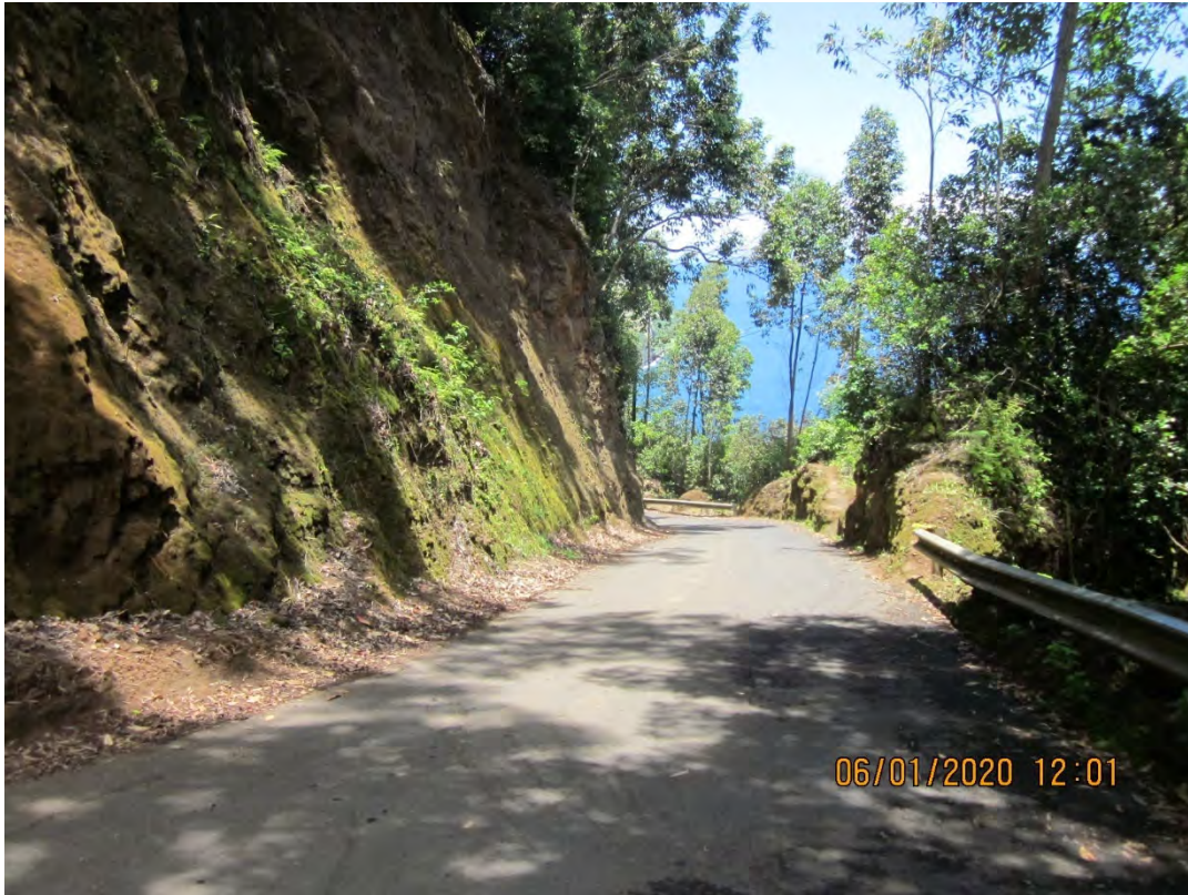
Photo 3. Transect F-W-02, Upper Section. Note the residual overhang upslope of road.
