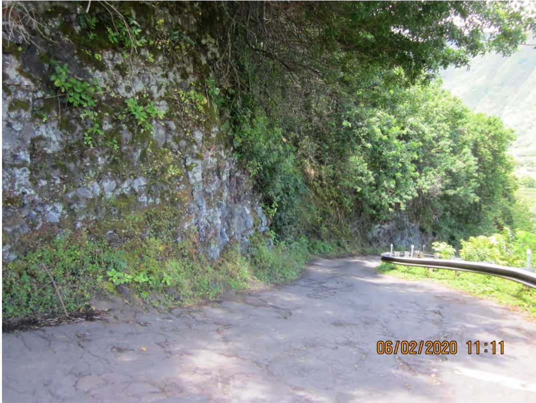
Photo 21. Transect F-W-10, Lower Section. Line-of-sight issues continue downhill.
