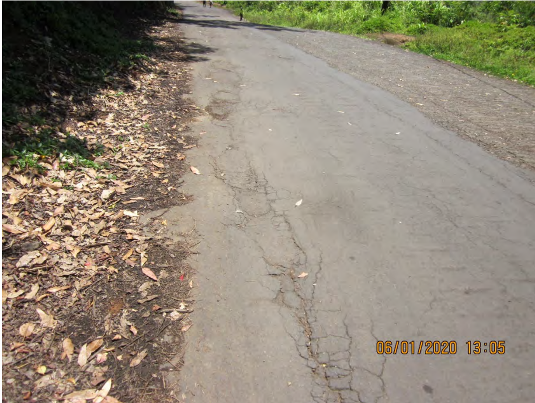
Photo 5. Transect F-W-03, Central Section Area. Note road wear and some potential rock strikes.
