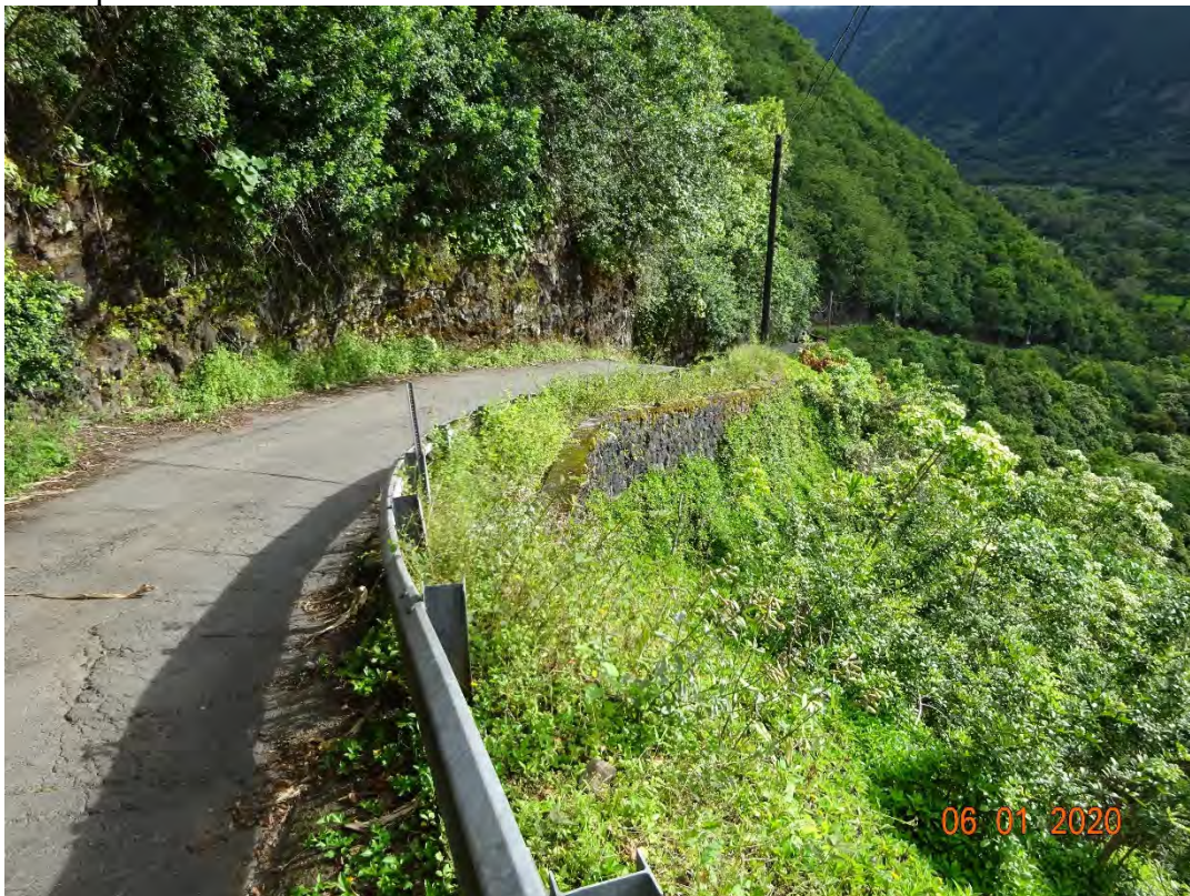
Photo 12. Transect F-W-05, Lower Section. Note rock retaining wall makai side of road.
