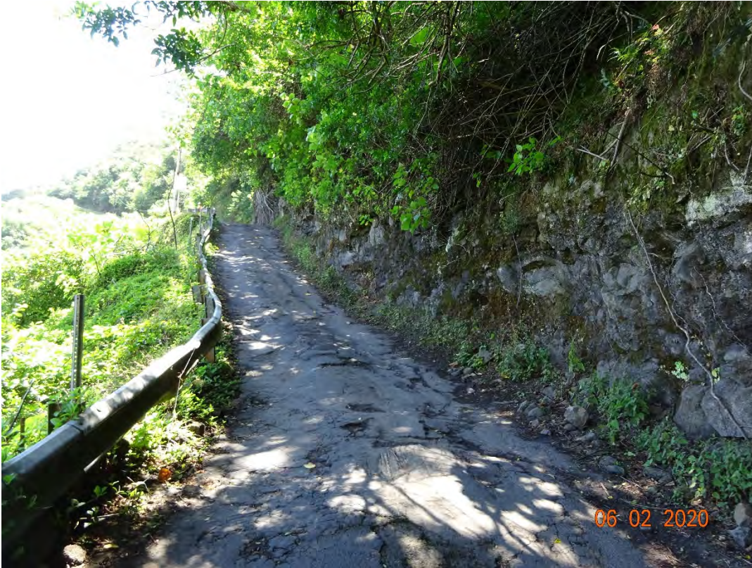
Photo 19. Transect F-W-08, Lower Section. Road narrows, Jointed Basalt with clinker zones observed upslope of road.
