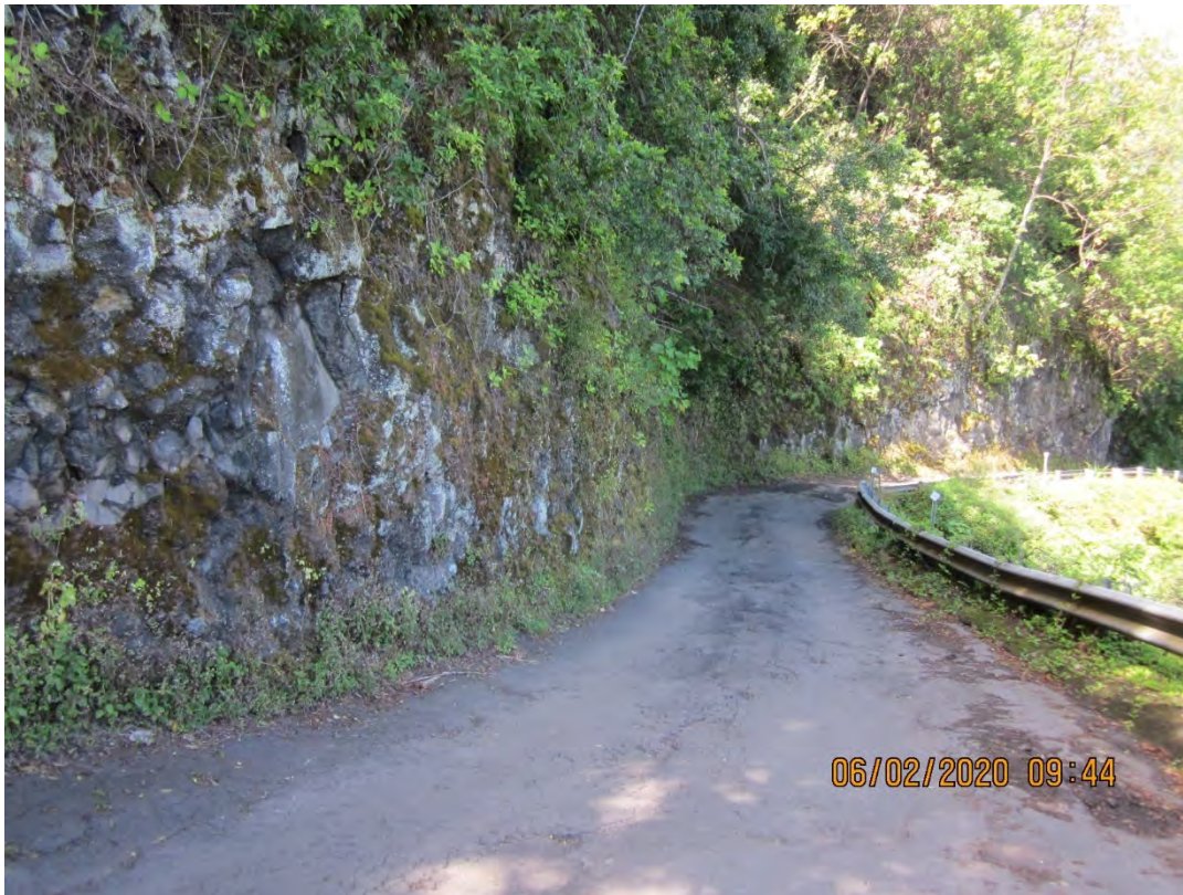
Photo 17. Transect F-W-07, Lower Section. Jointed Basalt outcrop with infilling.
