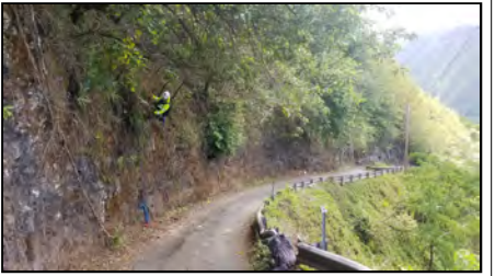
Slope Adjacent to Roadway
