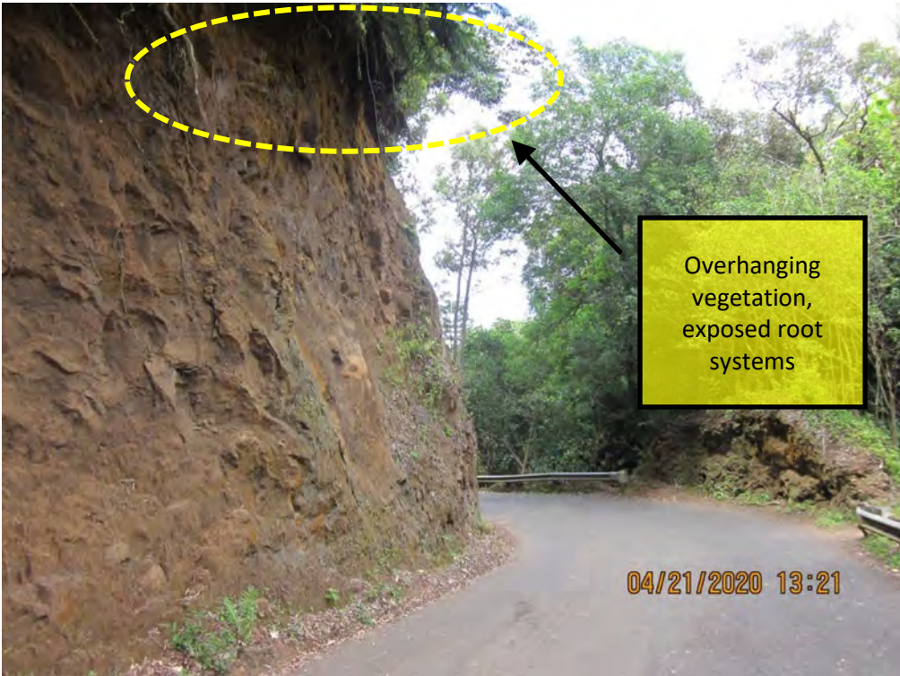
Photograph 4. Exposed soil of upslope road cut slope face. Note overhanging soil and vegetation.
