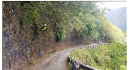
Slope Adjacent to Roadway
