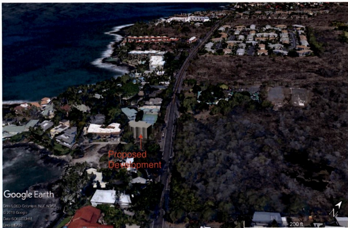
Figure 6a. Proposed development in relation to surrounding area. Ali'i Drive cuts roughly through the center of the frame northbound.
