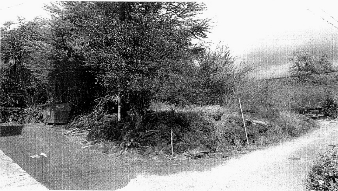
Photo 2 Overview of property from rear, view north-northeast.
