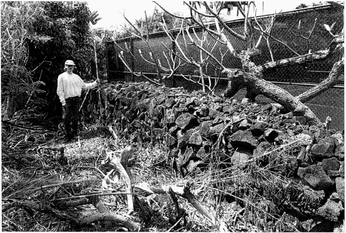
Photo 5 Intact portion of core-filled wall.
