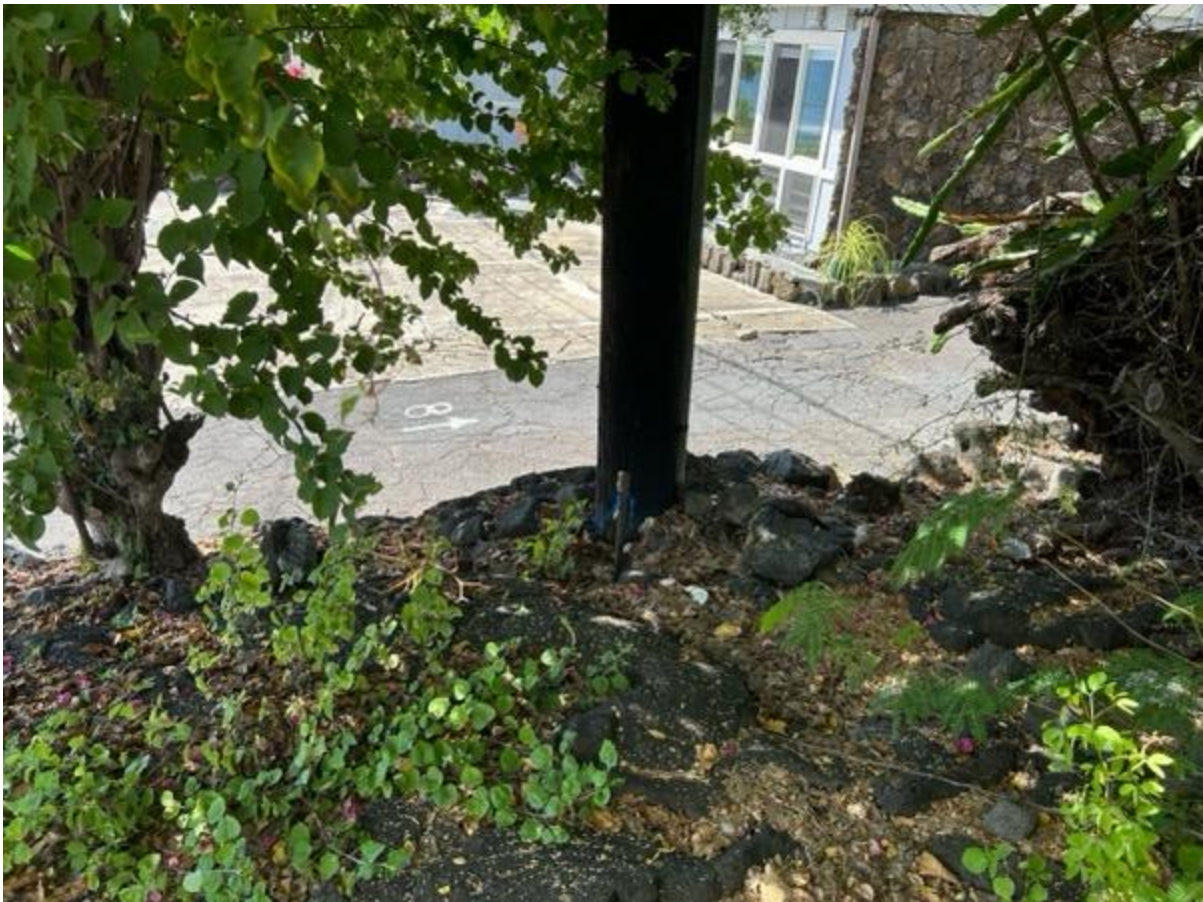
No. 2d: Boundary pin at base of power pole, Bo Bougainvillea tree to left
