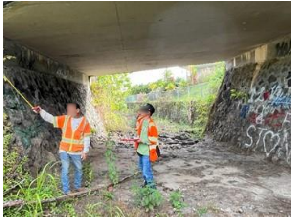
Bridge #24-3 Kupulau Road: Contracted Engineers conducting NBI inspections.
