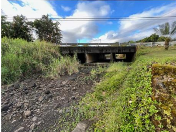
Bridge #24-4 Ho'aka Road Box Culvert: Vegetation on NBI box culvert.
