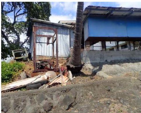
Structural encroachment on private property along the Pa'auau Channel.
