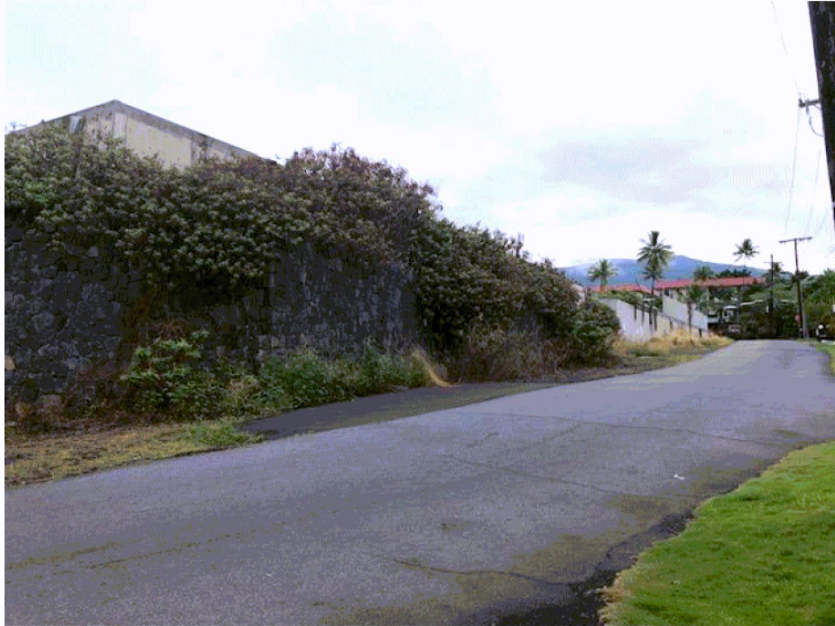
Photo 1: View of the property from the SW corner of Kahakai Road showing the slope of the proposed construction site. The applicants are proposing to construct their 40 foot tall building on top of this already-existing foundation and basement which are already over 20 feet tall along the west section of Kahakai Road.
