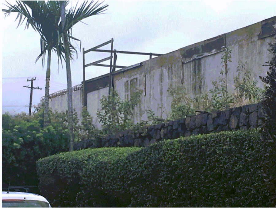
Photo 2: Existing structure as viewed from the west section of Kahakai Road. The applicants propose to build their 40-foot-tall building on top of this existing foundation and basement. The resultant building would measure ~65 feet tall on its west side along Kahakai Road.
