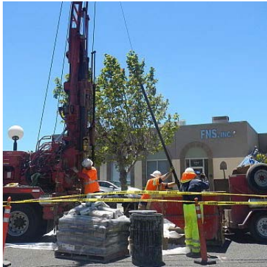
To expedite the investigation of PCE in groundwater, we used innovative tools including a cone penetrometer and a hydraulic profiling tool.
