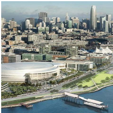
When contaminants were discovered during a ferry terminal project, Integral's engineering team provided a timely, cost-effective solution.
