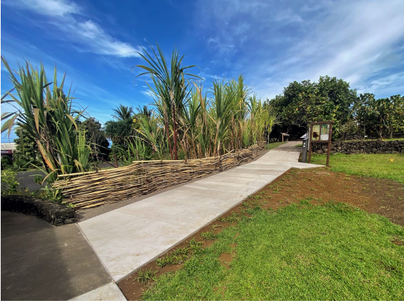
AGEG ADA entry path to Garden – with newly constructed bamboo fence with Hawaiian sugarcane, ko ,behind the fence.
