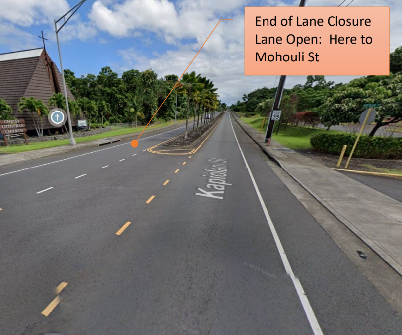
North End of Closure at Church and Hospice Facility
