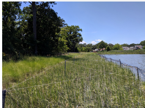
BC designed suitable, cost-effective sills to establish natural shorelines that protect and buffer the created wetland areas and shoreline banks from coastal flooding and erosion due to sea-level rise.
