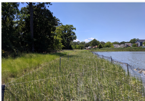
BC designed suitable, cost-effective sills to establish natural shorelines that protect and buffer the created wetland areas and shoreline banks from coastal flooding and erosion due to sea-level rise.
