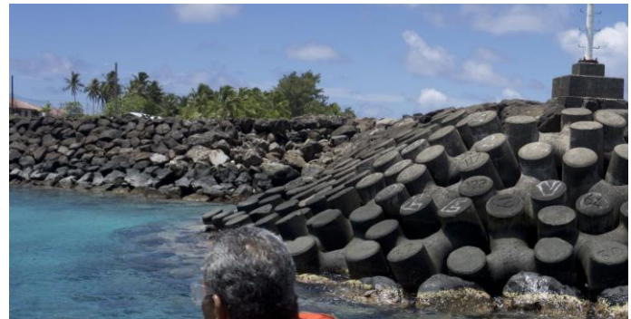
Sand on road indicating wave overtopping at Vatia Bay (top). Aunuu Harbor: damage to revetted mole at connection with stub breakwater from high wave event in July 2019 (middle). Shoreline erosion at Pago Pago port endangering options (right).
