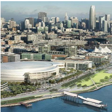
When contaminants were discovered during a ferry terminal project, Integral's engineering team provided a timely, cost-effective solution.
