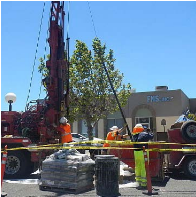
To expedite the investigation of PCE in groundwater, we used innovative tools including a cone penetrometer and a hydraulic profiling tool.
