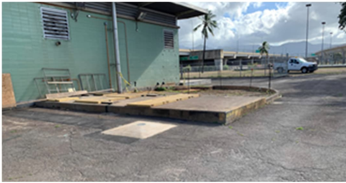
Pump Station and Wet Wells
