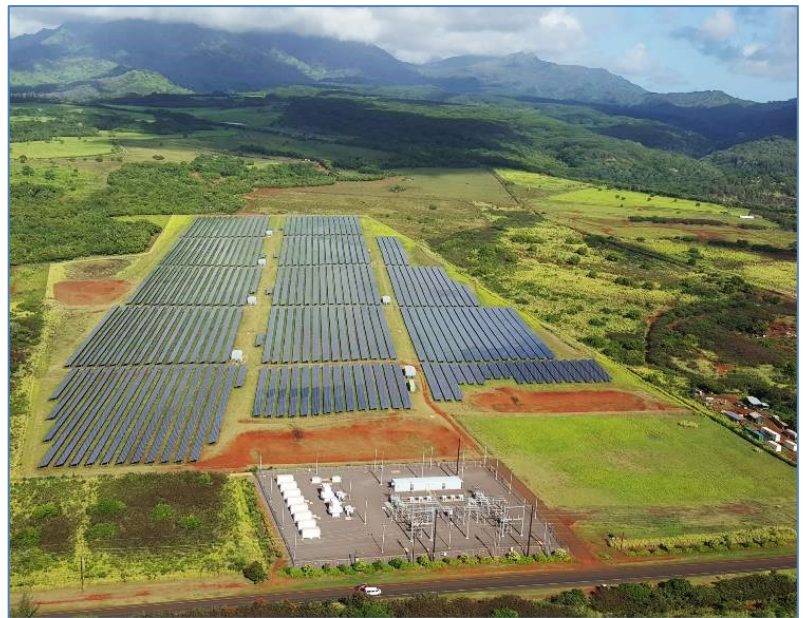
Completed Anahola Solar Project.
