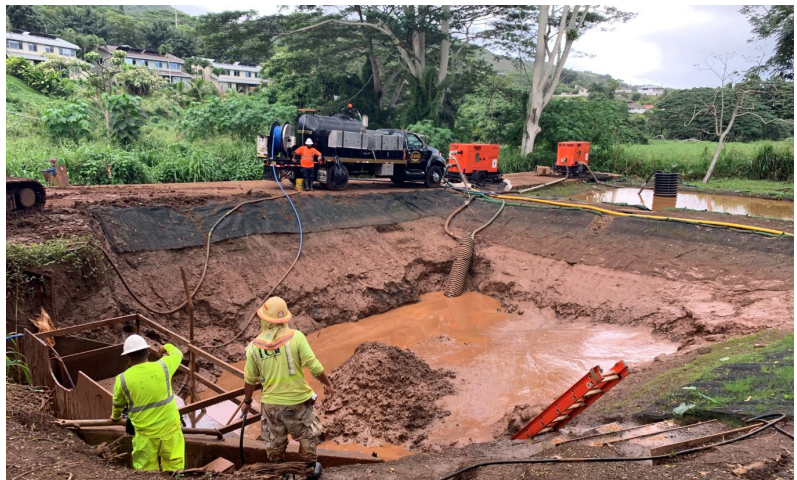
Basin (settling and dewatering) at outlet of culvert.
