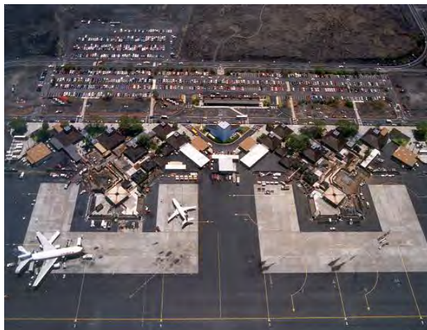
Various Construction Projects, Kona International Airport (1998-2009)
