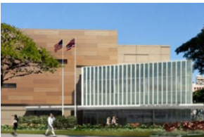
Honolulu Joint Traffic Management Center
