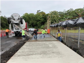
Kulani Correctional Facility Potable Water Supply
