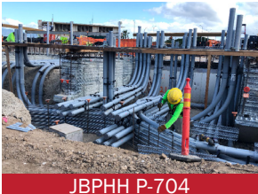
JBPHH P-704 Sewer Lift Station and Relief Sewer Lines
