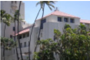
Honolulu City Hall Fire Alarm System Improvements
