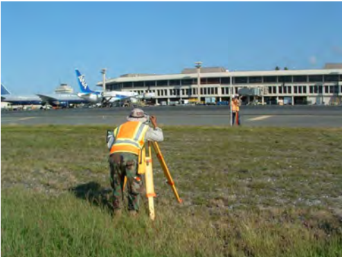
RMTC surveyors perform a topographic survey at the Daniel K. Inouye International Airport, Oahu.
