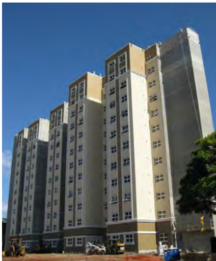
RMTC designed the civil sitework and obtained agency approvals for the construction of the new Frear Hall dormitory at the University of Hawaii at Manoa. It is certified LEED silver.
