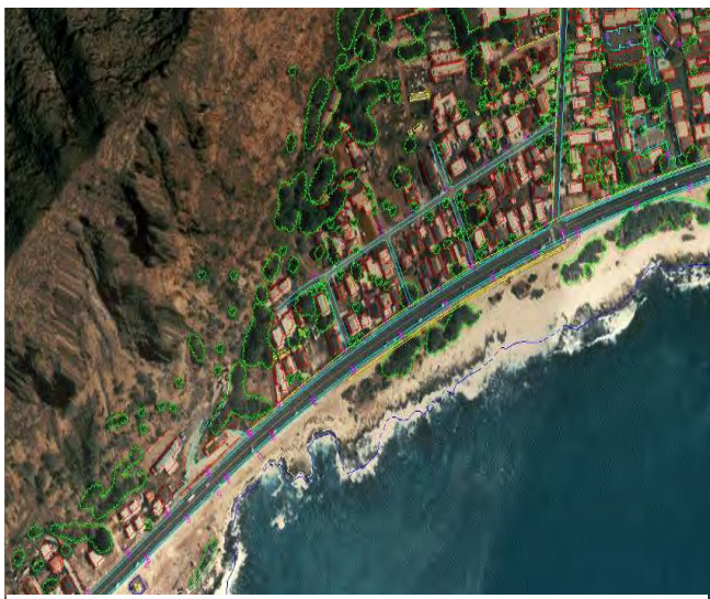
For the 17-mile Farrington Highway Safety Improvements project, RMTC engineers used aerial topographic surveys to support civil design.
