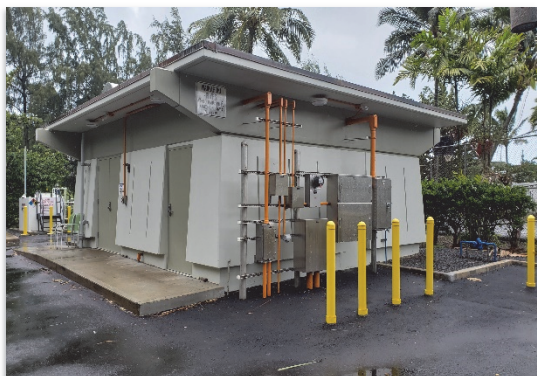
Refurbished pump station building with new fuel tank
