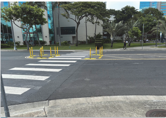
Existing crosswalk at Queen St/Waimanu St intersection
