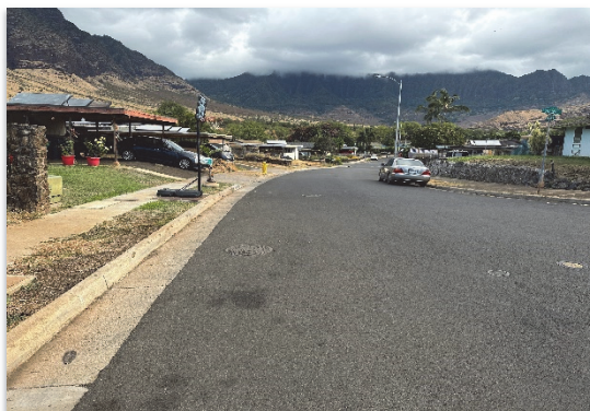
Pre-construction prior to sewer manhole rehabilitation and sewer line replacement
