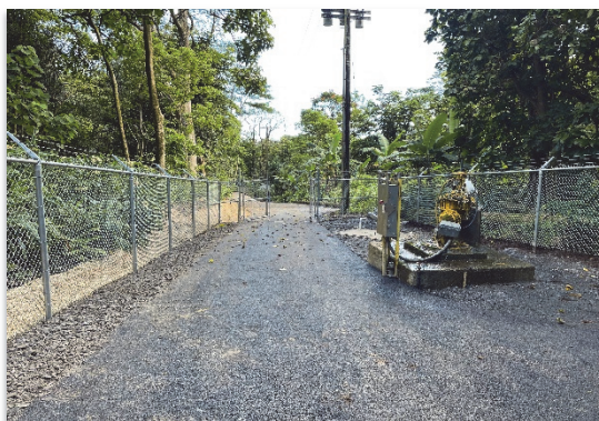
Reconstructed fencing and access road to the pump station
