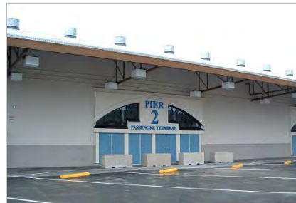
Pier 2 Cruise Terminal, Honolulu Harbor, Oahu (2006)
