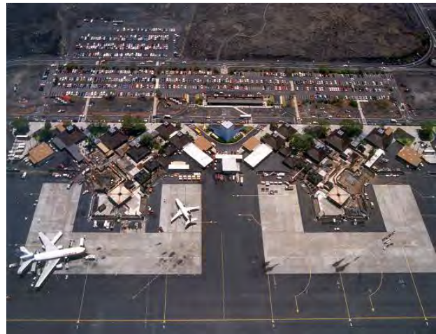
Various Construction Projects, Kona International Airport (1998-2009)
