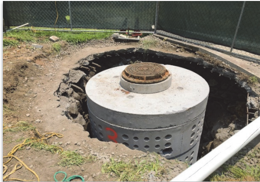
Seepage pit installation at Nani Olu
