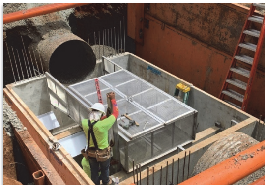
Hydrodynamic Separator being installed for stormwater quality improvements
