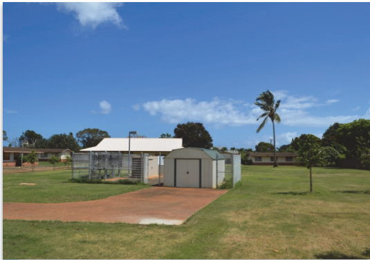
Completed treatment system site
