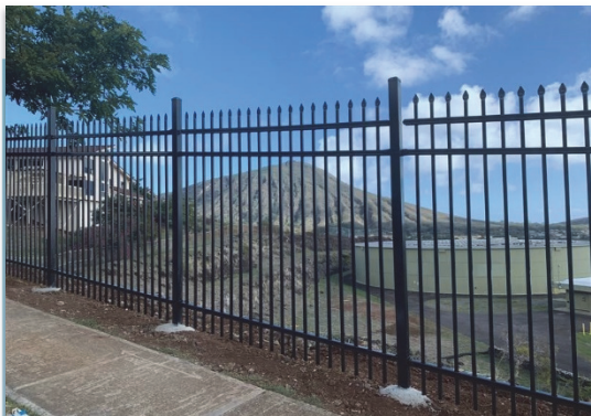
Palisade fencing installation at Mariner's Ridge 170 Reservoir & Booster 1
