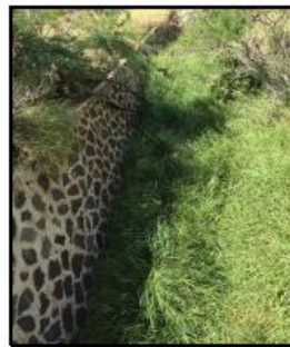
Parapet for target area.
