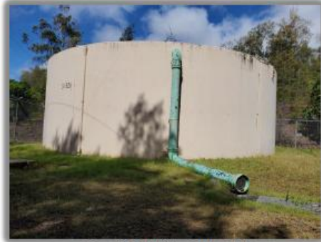
Camp Smith Water Tank S-326
