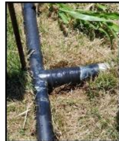
Repaired Sprinkler piping at Tripler Landfill, TAMC-02
