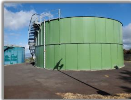
Red Hill Water Tank
