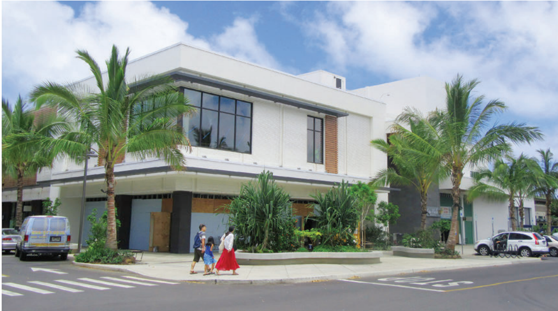
Building entry along Lau Hala Lane
