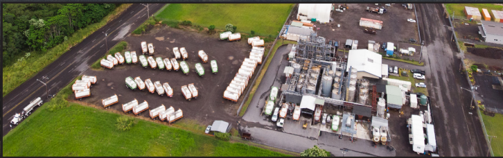
Shipman Industrial Park, Keaau, Hawaii Civil engineering for the third largest industrial park in the state.
