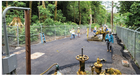
Waihole Well Site Repaired
