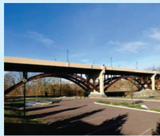
State Route 113, Gay Street Bridge
