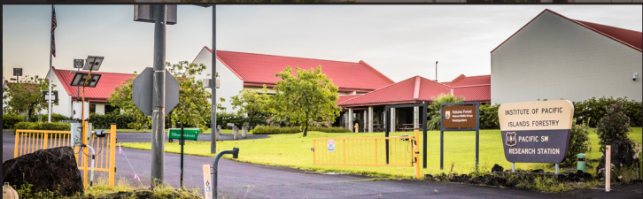
Institute of Pacific Islands Forestry, Hilo, Hawaii Civil site development for this center for research and technology transfer.
