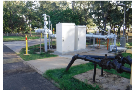
Wailua upgraded pump station site
