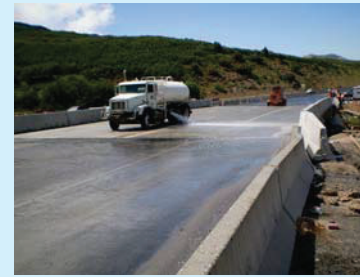
New bridge deck on Interstate 80
