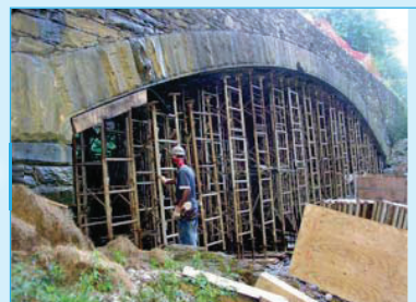
Installation of supports under masonry arch
