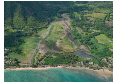
Punaluu Stream Restoration Project at Substantial Completion
