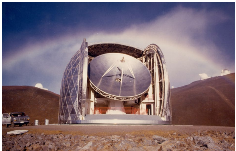
CSO with dome open.
