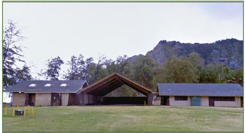
Southern view of pavilion before removal.
