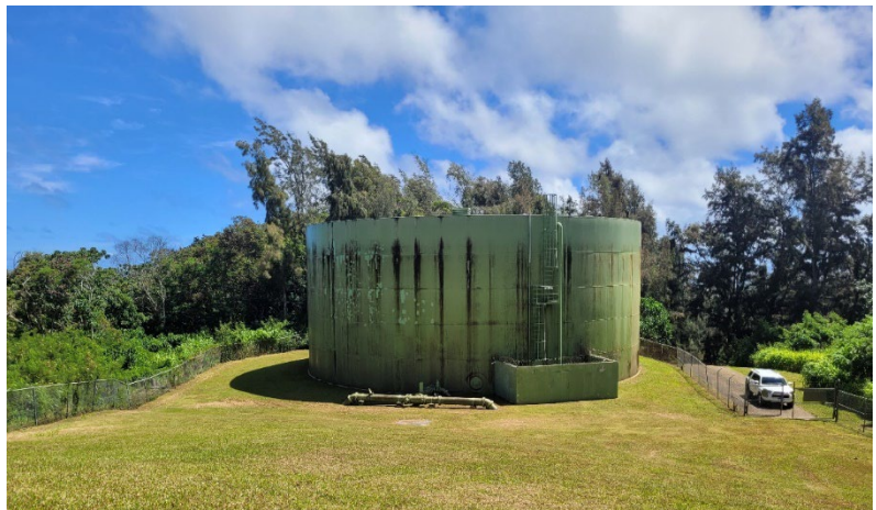
LWC tank and well site.
